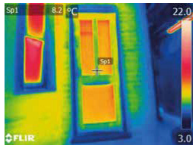
Traditional timber panelled door
